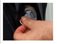
6. Replace the cap on the valve, before covering it with the Velcro sleeve to maintain a tidier external aesthetic. Repeat steps #3 to #6 with the three bedroom annexe tubes.
